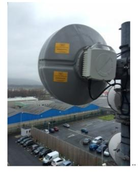
Antenna De-ICE System. The formation of ice and snowfall, especially on parabolic antennas, is a major cause in loss of signal transmission and reception during winter months. Faini Telecommunication System collaborating with experienced heating manufacturer in order to provide a reliable De-ICE system keeping the antennas operational in the most severest of weather conditions and thus preventing interference and costly down time.
